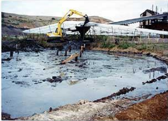
Removing sludge from storage pond
