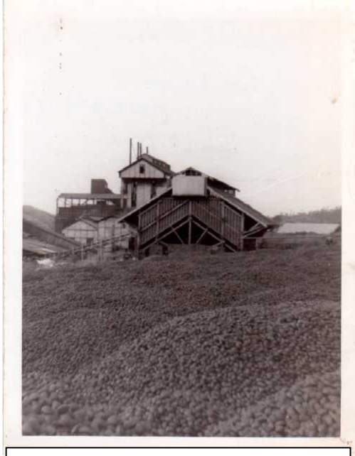
The carbonisation plant, surrounded by piles of carbonettes, ready to be sold as household fuel. (2004.192.1)
