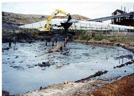
Removing sludge from storage pond
